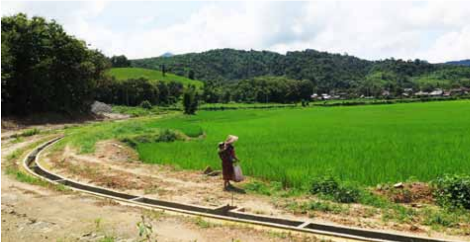
New canal systems were installed as part of the irrigation scheme in Kay district, Vientiane province
