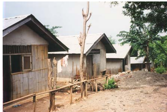
Fig Abandoned Houses in Nangahure, the occupants moved back to their original Wuring village, March 2001.
