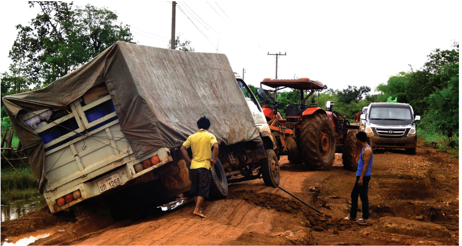
Typhoons in Khammouane province cause economic losses, as well as physical damage.
