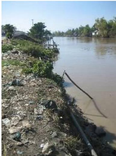
*Figure 1: Bridge 10 - Illustration of river- bank erosion*
