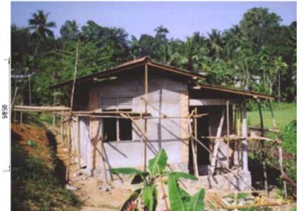
The actual construction at the site
