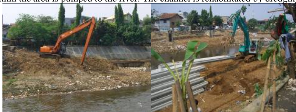
Figure 6. River Protection and Rehabilitation in Kebon Baru Area
