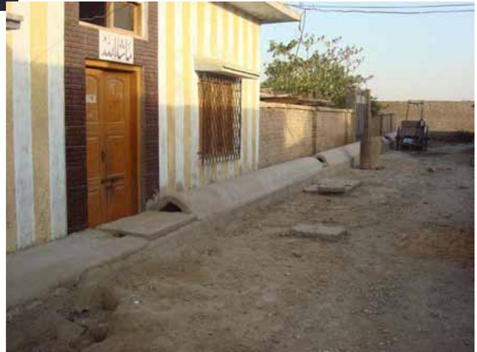
Aliabad after Drainage
