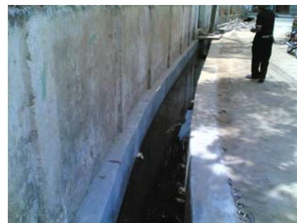
Improved Drainage, Jalalabad Ward
