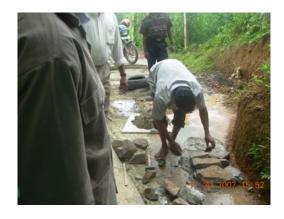
Another suggested structural mitigation project under PROMISE is to build proper drainage system as a solution for the road inundation during the heavy rain. As a first step of our second mitigation project we took the level measurements along the road with the support of the technical officer and calculated cost breakup.
