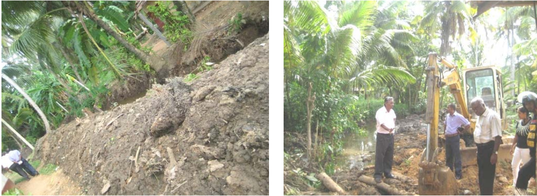
Progress of the Mitigation Activities
