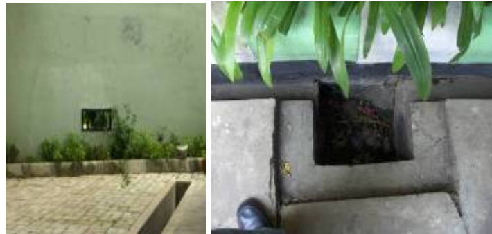
Figure 2. School DRR Initiatives on : Holes at the wall fences around the school and drainage system connected to Ciliwung River
