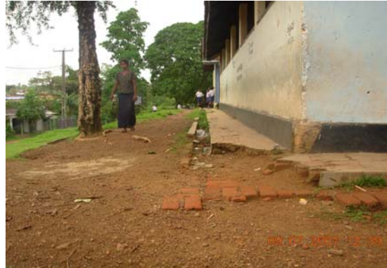
Soil Erosion problem and broken Drainage lines of Nagoda School, Kalutara
