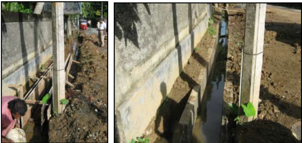
Figure 07: Construction of New Drainage
