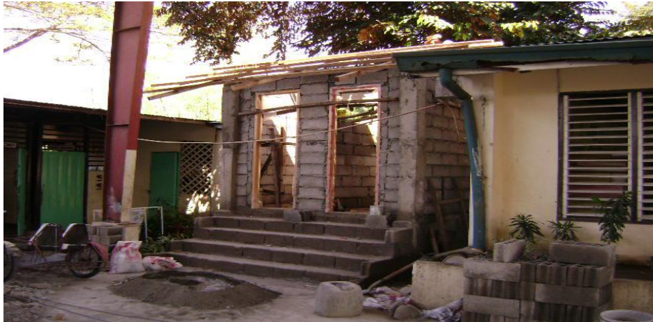
A barangay elevates its community toilet as part of its structural mitigation efforts
