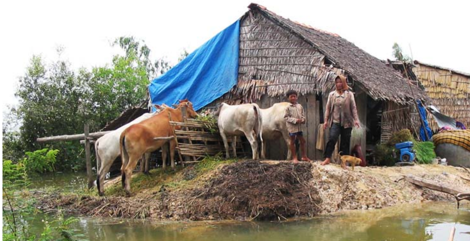
Elevation of homesteads and roads above maximum recorded flood level in Bangladesh, called flood proofing
