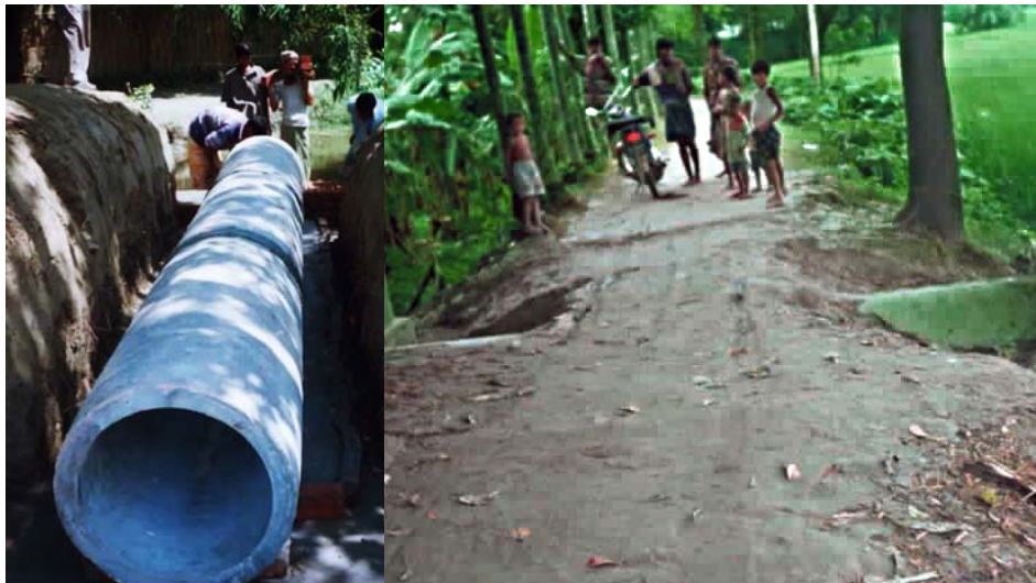
Structural mitigation for floods also ensures adequate size of culverts, and other drainage devices built to control floodwaters, and bridges to ensure access over flooded areas. Drainage is a major problem in the floodplains of Bangladesh. Improvements to old drainage systems and introduction of drainage pipes in areas experiencing population growth can reduce the level and duration of inundation. A minor structural intervention in a community-based initiative in Bangladesh has lessened the severity of flooding in these growing urban environments.
