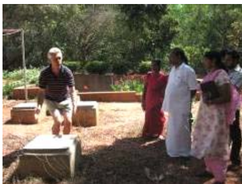
DEWATS at Auroville
