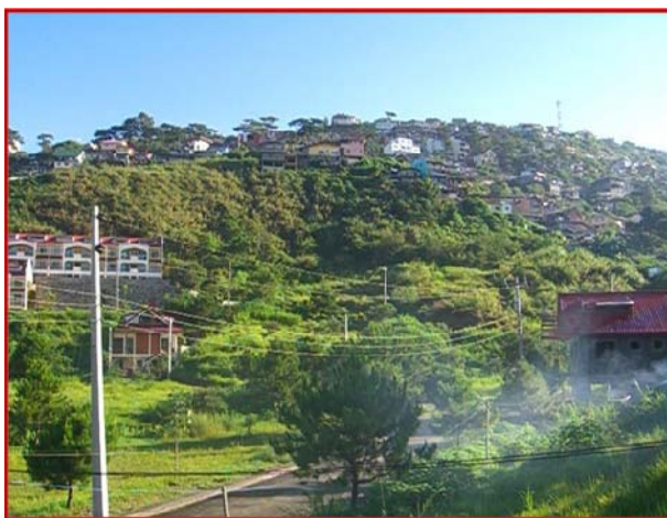
Figure 10: The San Luis Landslide Site, a view from the base hill.
