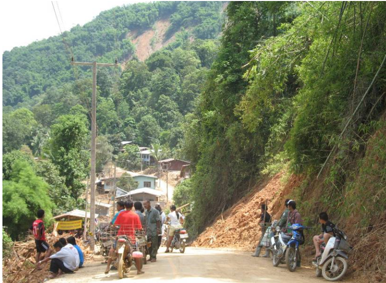
Figure 4. Poor practices of settlement: construction of houses on hill slope
