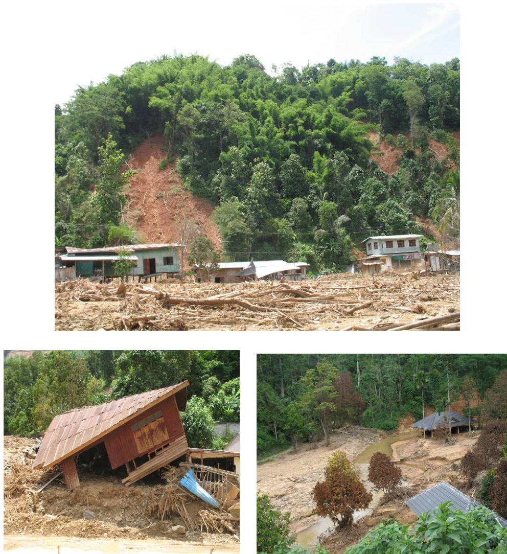
Figure 5. The destruction of traditional houses due to slope failures (above) and its proximity to the streams.
